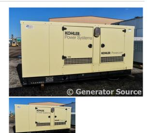
**Description:** Kohler 150 kW Natural Gas Generator Model #: 150REZGC Serial #: SGM329XG4 Year 2014, 158 Hours, 277/480 Volt, 3 Phase, Sound Attenuated Enclosure
