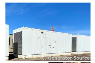
**Description:** Cummins 1750 kW Diesel Generator Model #: DQKB5568336 Serial #: I020418328 Year 2002, Less than 500 Hours, 480 Volt, 3 Phase, Sound Attenuated Enclosure with Base Fuel Tank
