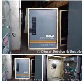
Description: Kohler 104 Amp Automatic Transfer Switch, Model #: K166541-0104, Serial #: 0698108, 480 Volt, 3 Phase, Nema 1
