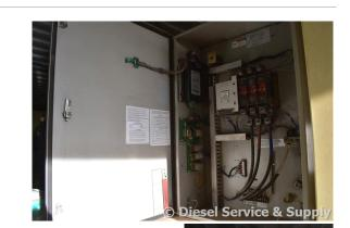
Description: Generac 150 Amp ATS Model #: 10921470100 Serial #: 99457 3 Phase, 208 Volt, Nema 3, 3 Pole, 4 Wire
